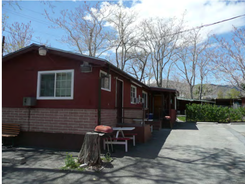
Motel Building (located south of Lodge building)
