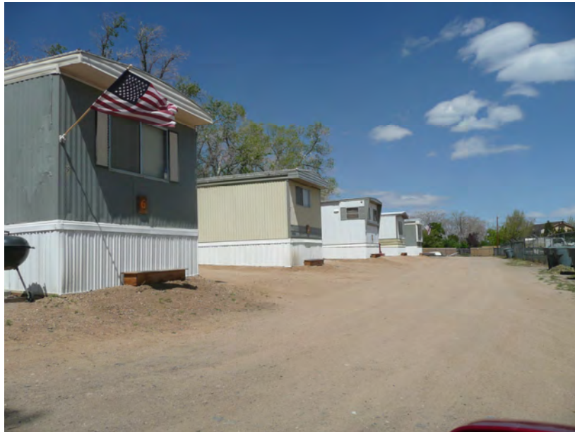
Modular Motel Units
