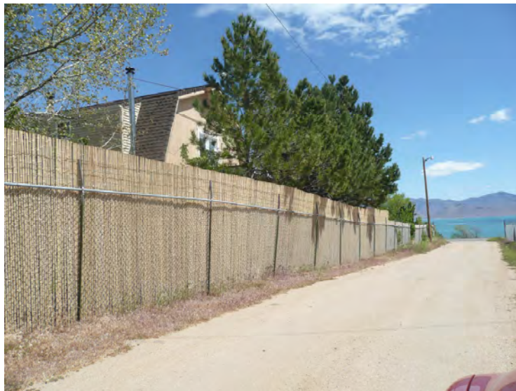
Figure 2-14 – Existing Permitted Screen Fence
