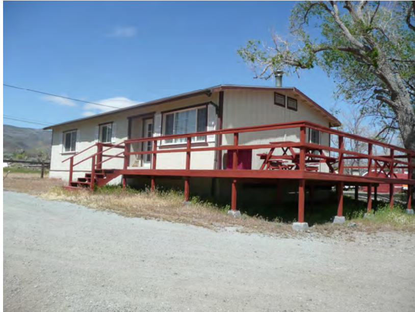
Modular Motel Units
