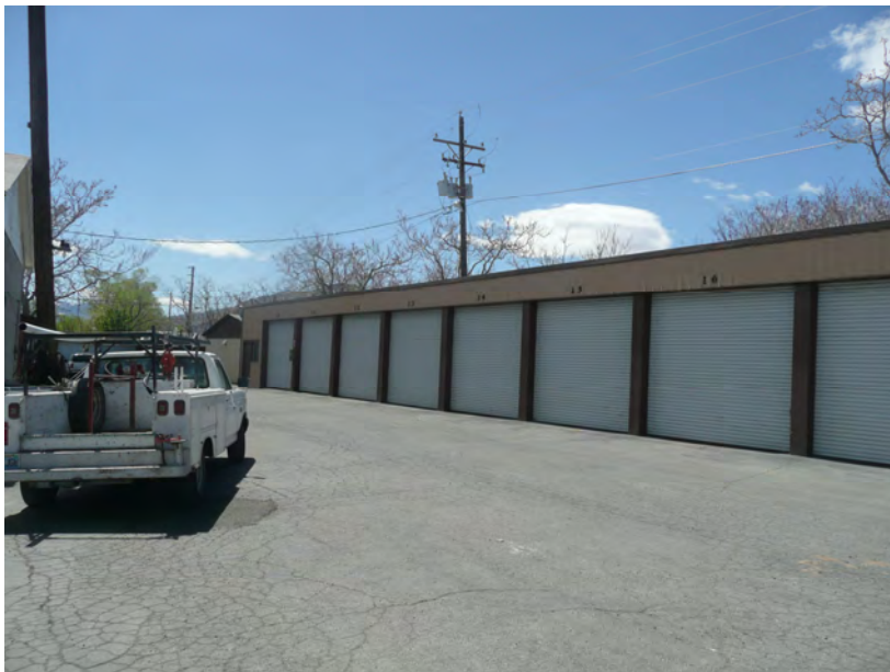
Enclosed Storage (located behind Lodge/Marine Shop)
