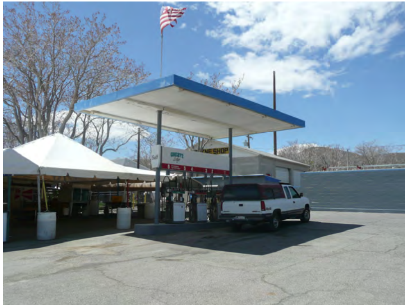
Gas Station (located on northern side of Lodge building)
